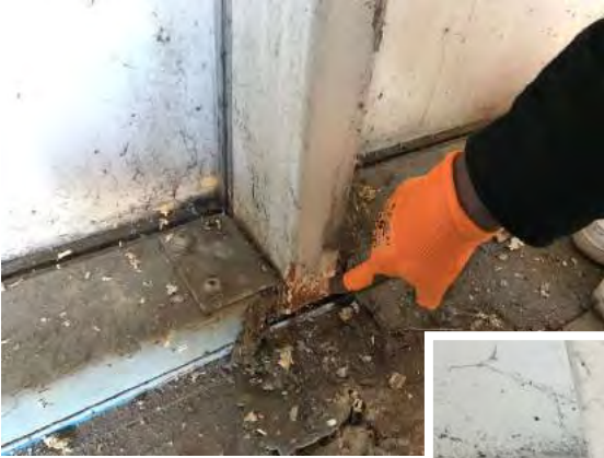
Pointing out how humidity has affected the building's facade
