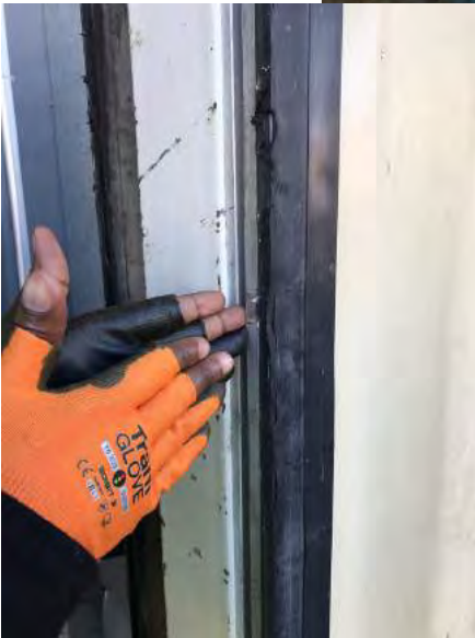
Demonstrating how the new double glazing unit fits into the profile - one glass pane is longer allowing it to fit within the existing profile
