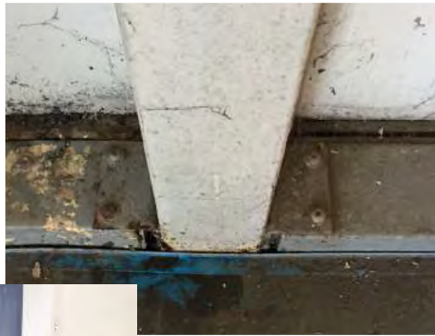
Demonstrating how the new double glazing unit fits into the profile - one glass pane is longer allowing it to fit within the existing profile
