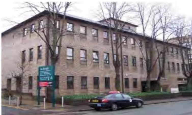
Daedalus house at 30 Station Road
