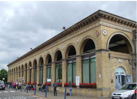
Cambridge station brickwork facade
