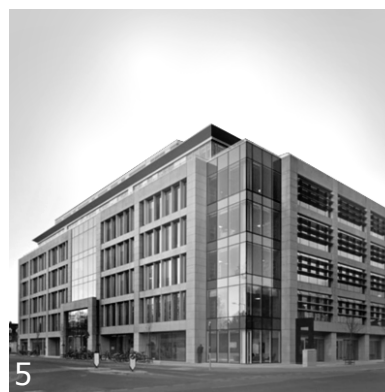
5 Microsoft's office is CB1 redevelopment first completed building. It was completed in 2012.
