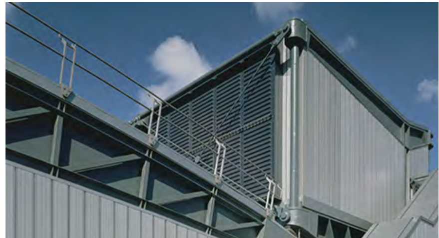
Close up detail of roof ( www.grimshaw.global )
