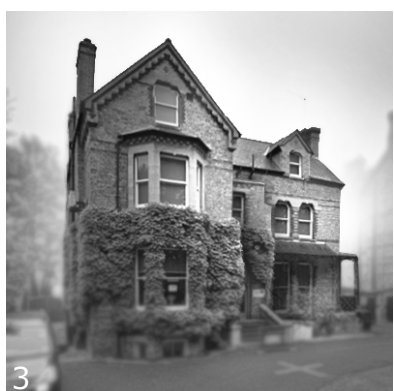
3 There are various Victorian houses still remaining. They were built in 1874 and designed by Richard Rowe
