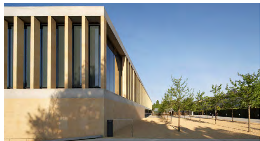
External facade ( www.stantonwilliams.com )
